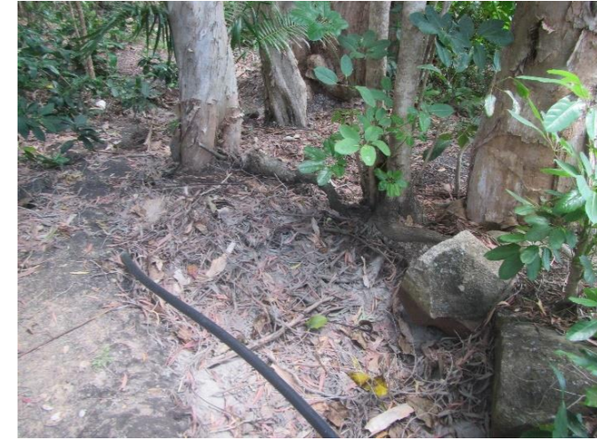
Plate 12: Pipe outlet at upstream ill-defined swale depression within the project site
