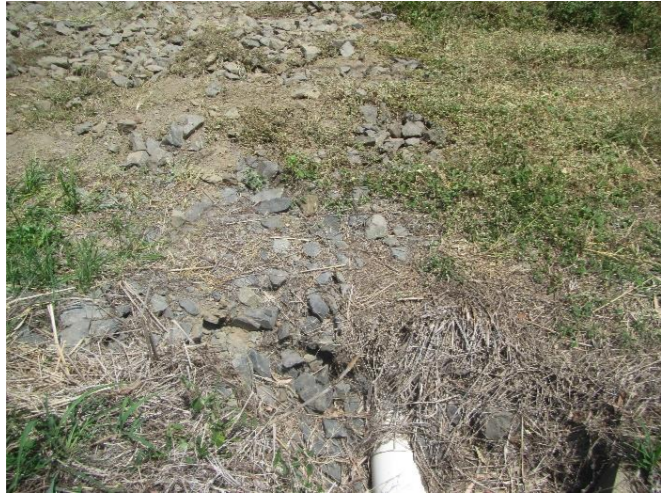
Plate 10: Drainage feature headwater origin at rock filtration stormwater diversion on southern side of Savage Street
