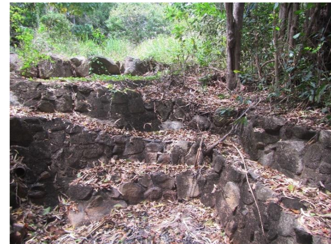
Plate 15: Steeply terraced rock wall (2 m high) is a waterway barrier for fish passage (facing upstream with swale depression above wall)
